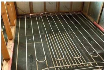
Homes at Fairlie being constructed to 'future home' standards, with under-floor heating, enhanced insulation, triple glazing and powered by air-source heat pumps. The lessons from this development will inform future schemes.
